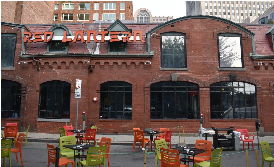
Photo 3. East half of 39-45 Stanhope Street facade, looking north.
