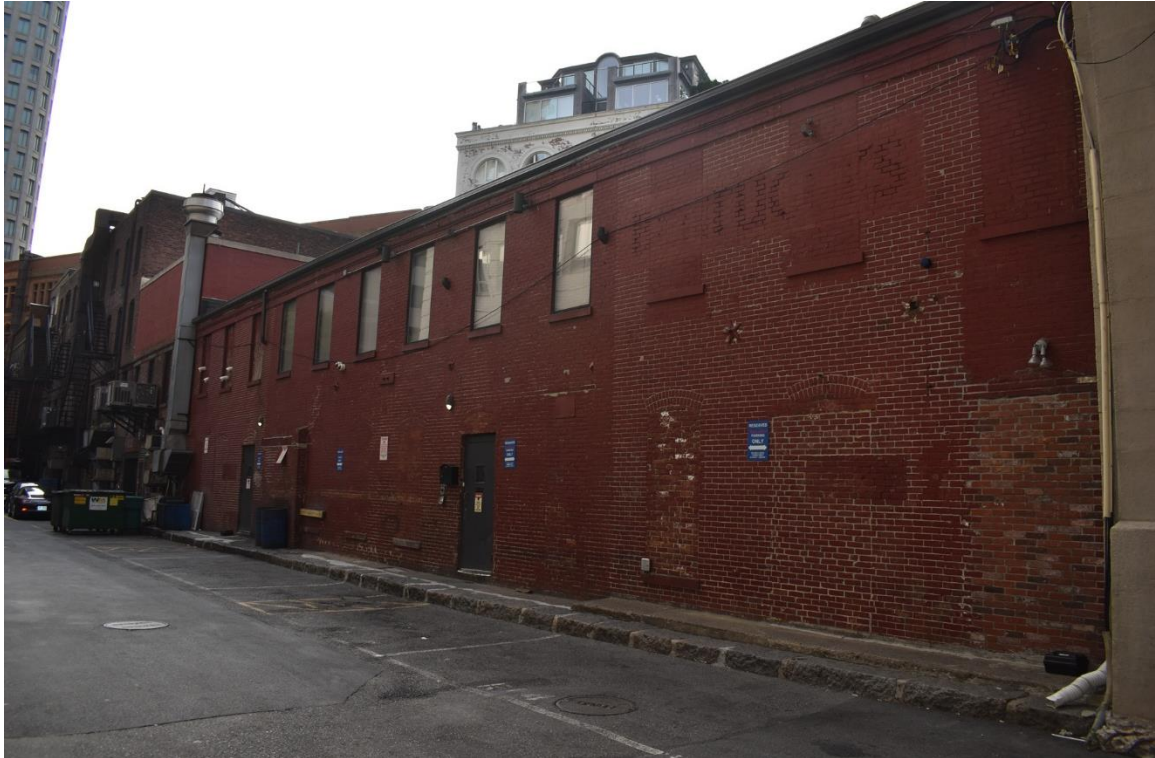
Photo 10. 39–45 Stanhope Street rear elevation, looking east.
