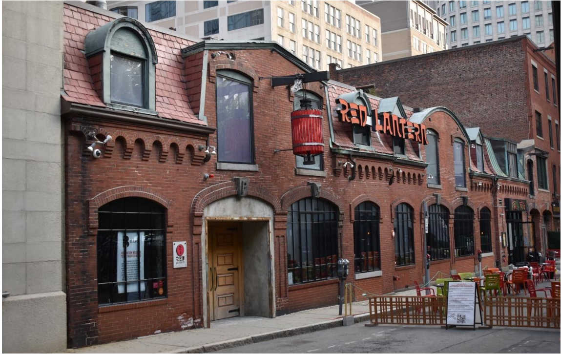
Photo 1. 39-45 Stanhope Street facade (south elevation), looking northeast.
